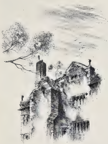
No. 4.—A Chimney, East Front, Livesey Hall.
